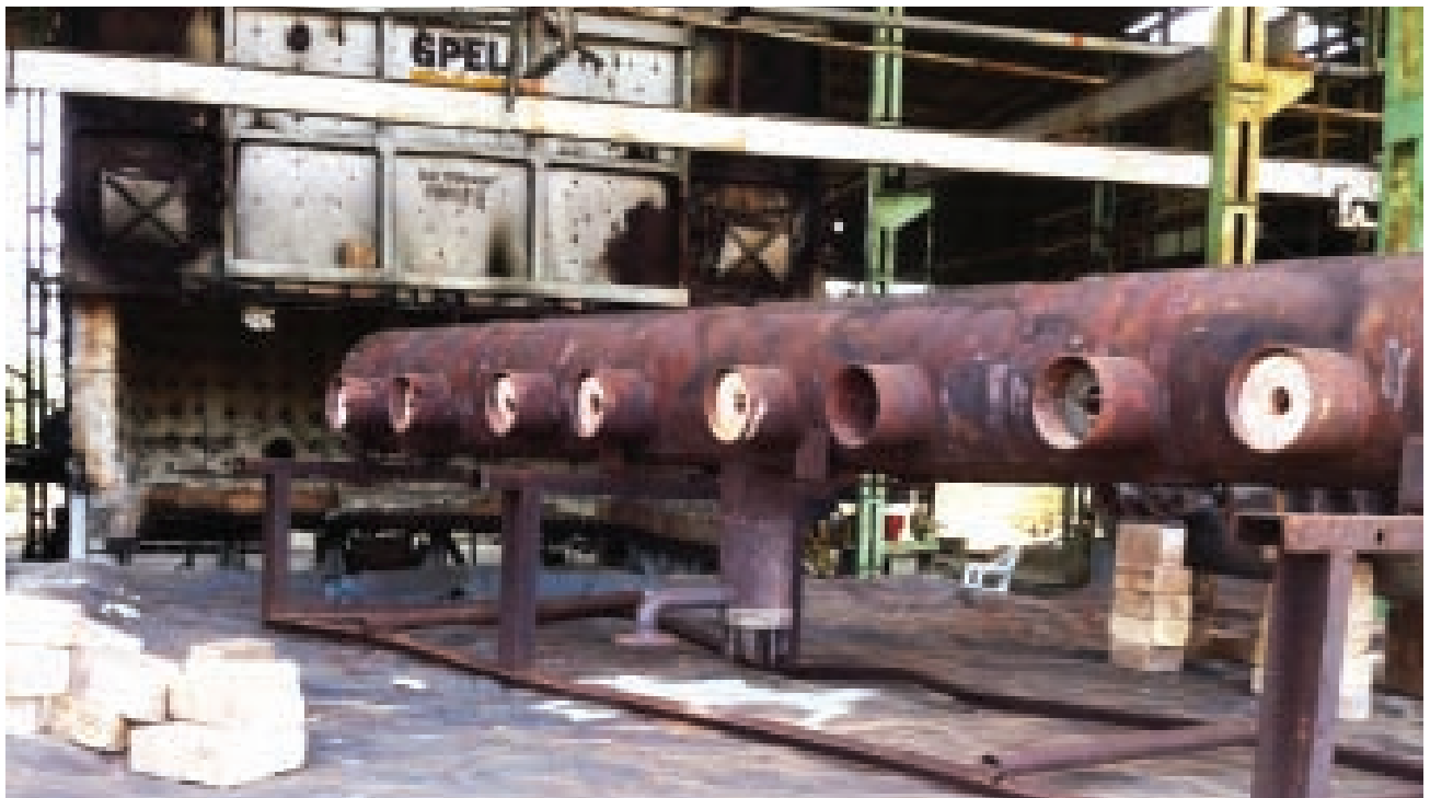
PWHT of 12 meters Length Vessel
